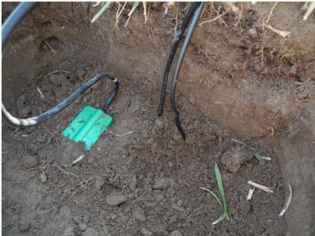
Figure 2. Installation of soil moisture sensing probes at multiple depths.
